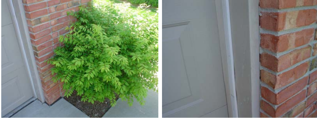
Trim Bushes - Caulk around door
